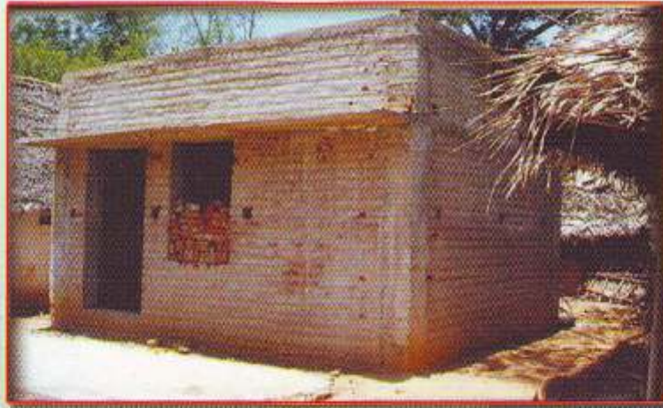
FLOOD RELIEF - HOUSE CONSTRUCTION NEARING COMPLETION AT NEDUNTHERU
